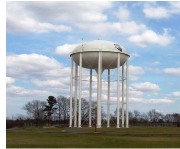
Pinedale Road Water Tank
