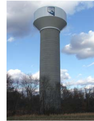
Pepper Road Water Tank
